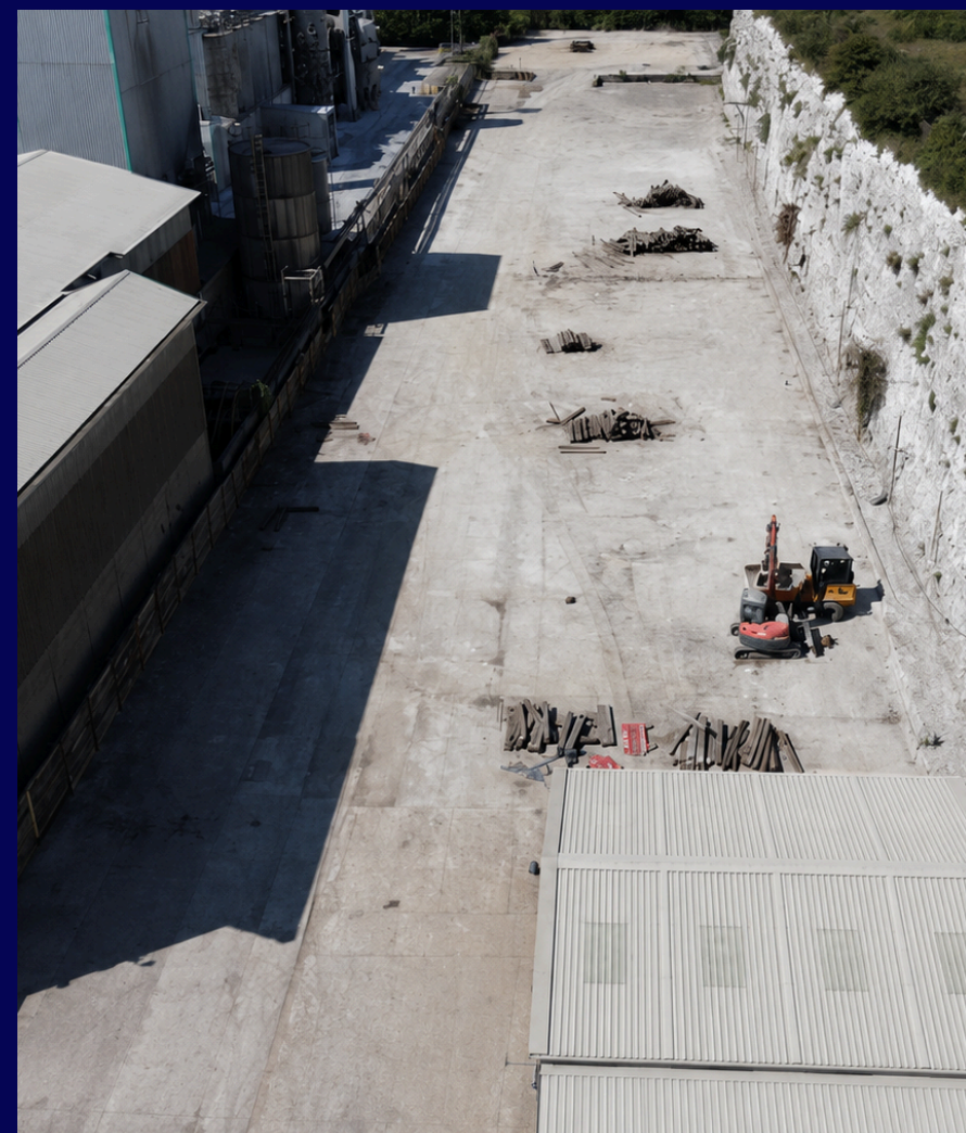
Yard clearance in progress
