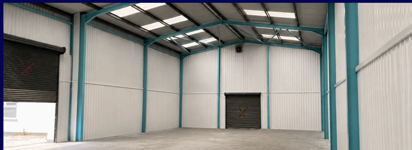
Refurbished warehouse interior
