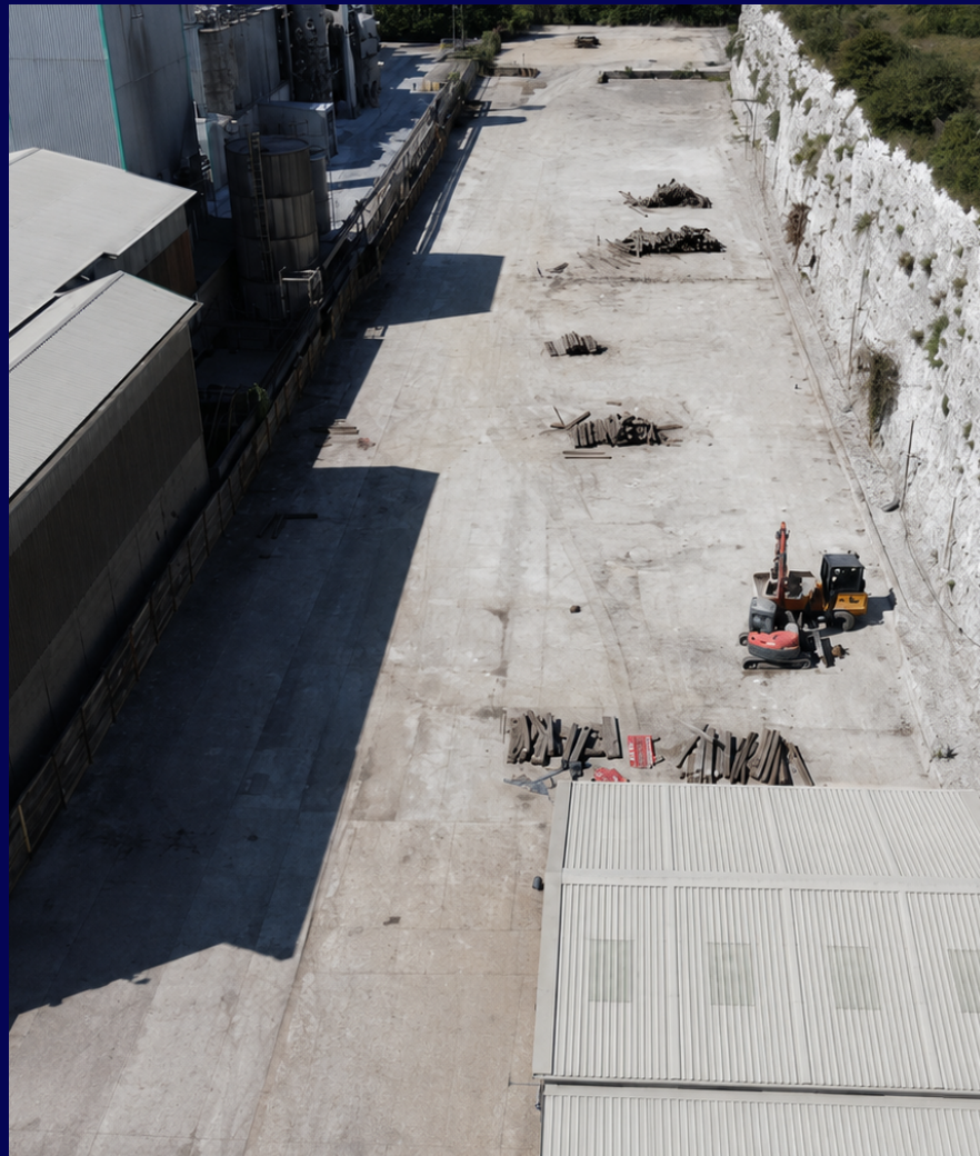
Yard clearance in progress
