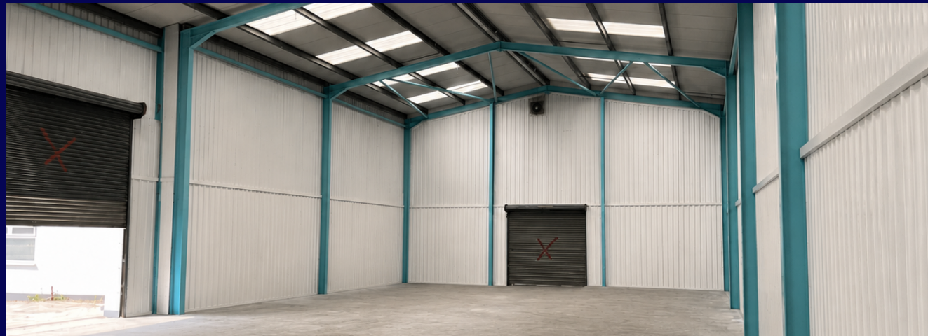
Refurbished warehouse interior
